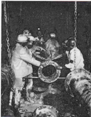
Cleaning up after the valves were closed: the extension pipes on the valves being removed prior to the blank flanges being bolted on.
