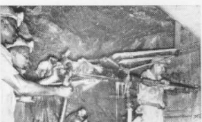
A cementation pipe in a plug being drilled open to allow tightening of the plug.
